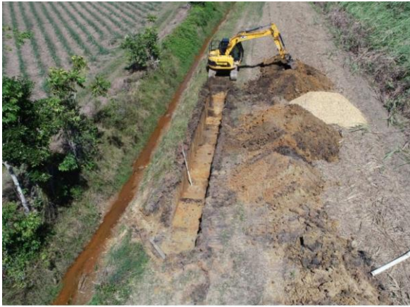
Trenches are filled with woodchips to build a bioreactor, where microbes operating in an anaerobic environment remove nitrates that would otherwise flow into local rivers. (Supplied: Terrain NRM)
